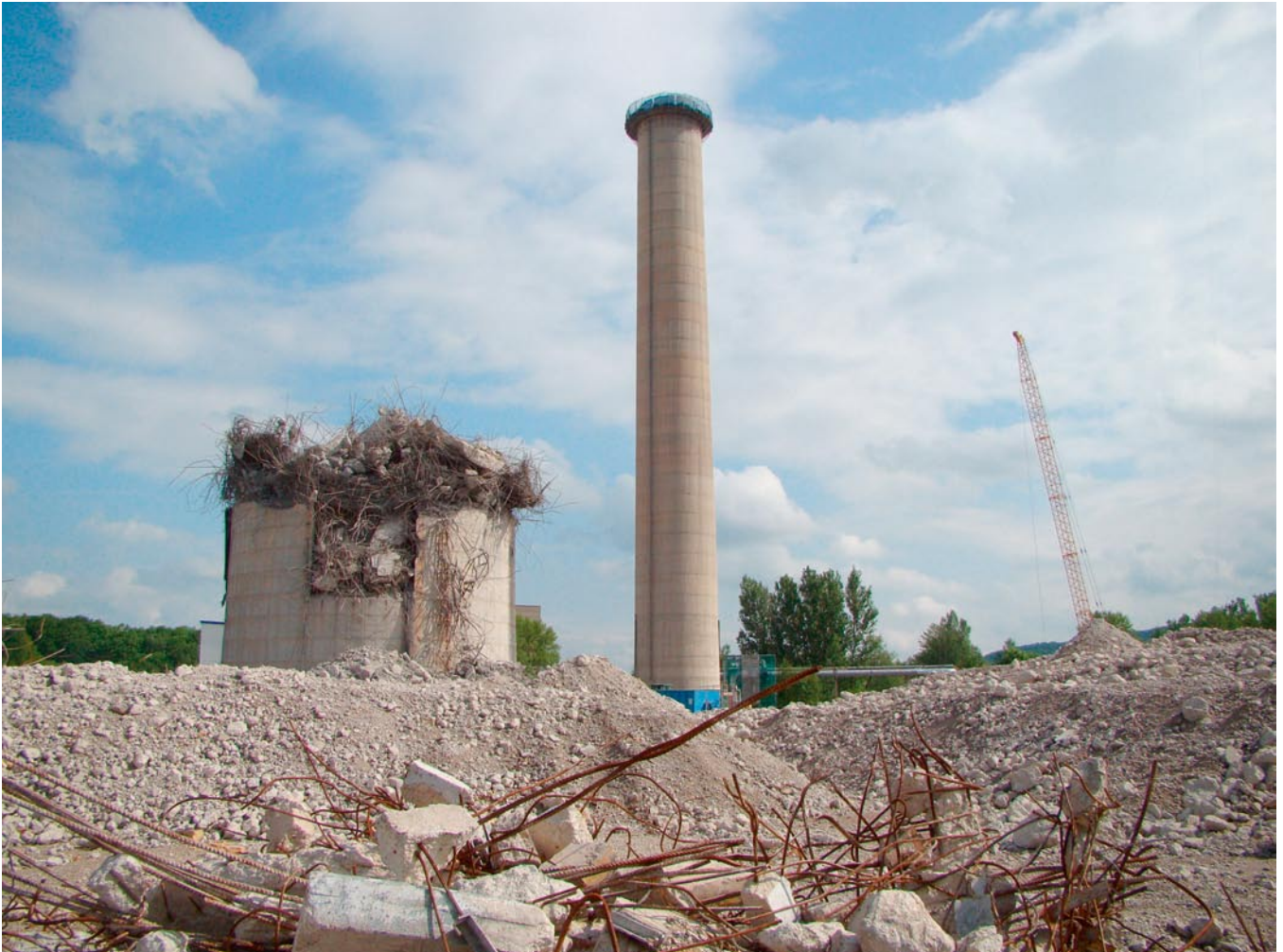
Schornstein-Abbruch in Gera/Deutschland • Demolition of roofs in Gera/Germany
